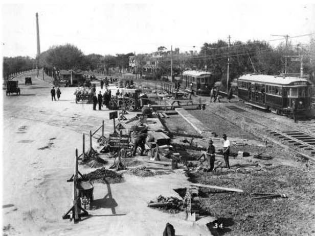
St Kilda Road electrification c 1926 at Domain Rd. Inbound W class to North Coburg leads another W. Chimney stack of engine house in left background.
