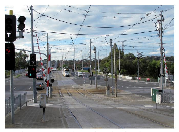
Tramway level crossing at Burke Road Gardiner on 19 April 2012, looking north. A Z3 class tram is waiting at the traffic lights before proceeding to the city, while the tramway 'T' traffic lights that replaced the original disc signals are prominent on the left. Note the catch point in the foreground. This scene is now disappearing under the works of the level crossing replacement project. Photograph by Mal Rowe.
