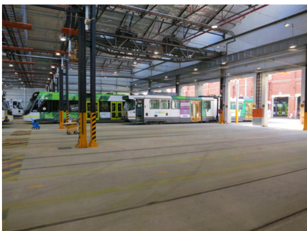
Inside one of the cavernous running sheds
