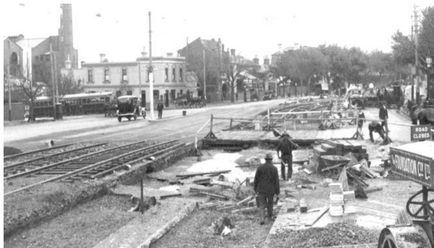
Looking north showing disconnected Domain Rd track (front right) and W class tram in Park St, South Melbourne (left) using diversionary route to Swanston St. Photo: SLV, handle.slv.vic.gov.au/10381/336839
