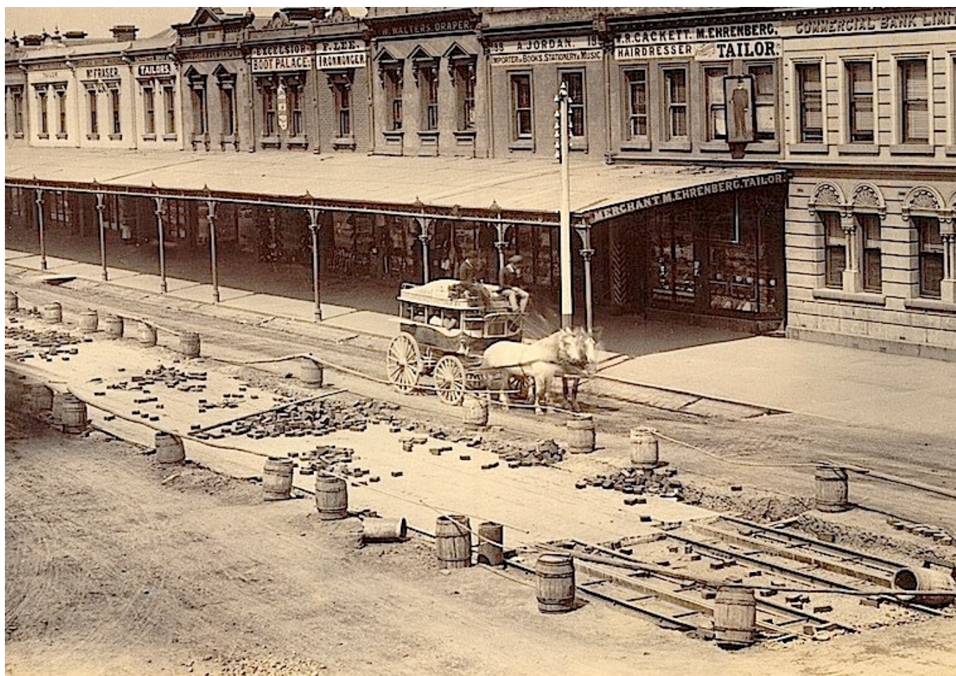
Cable tramway construction in Clarendon St, South Melbourne at the corner of Bank St looking south (1888).
