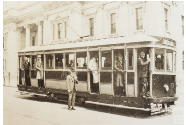
Q class 173 in front of the Prahran Town Hall – the first electric tram after the conversion. (1926)
