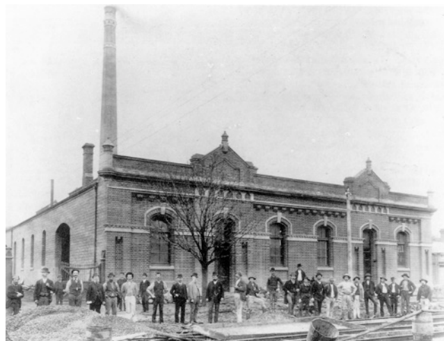
The newly built South Melbourne engine house in Sandridge Rd (now City Rd) with track construction in progress (1889). Photo: Jack Cranston collection
