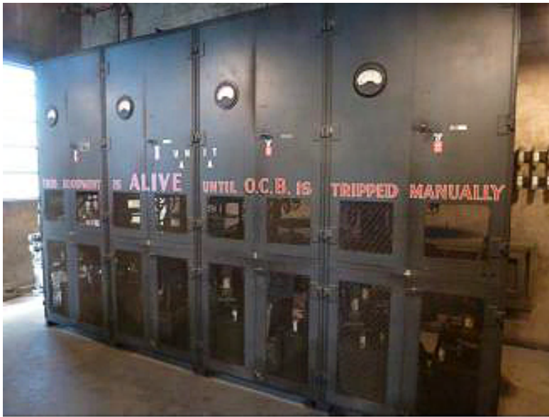
ABOVE: Bank of four cabinets inside the Brunswick West Substation that each contain a mercury-arc rectifier. RIGHT: An activated mercury-arc rectifier inside one of the cabinets (2019).
