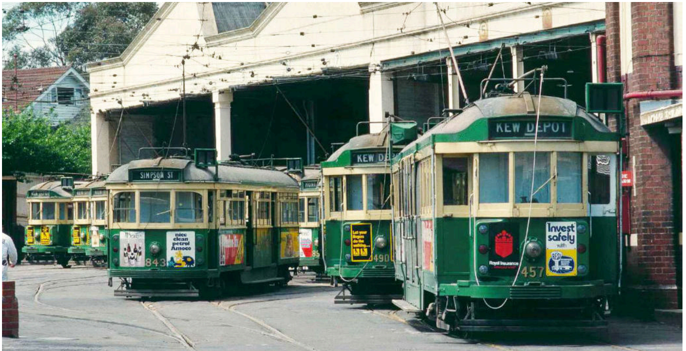
ABOVE: Kew Depot track fan and running shed (1975).
