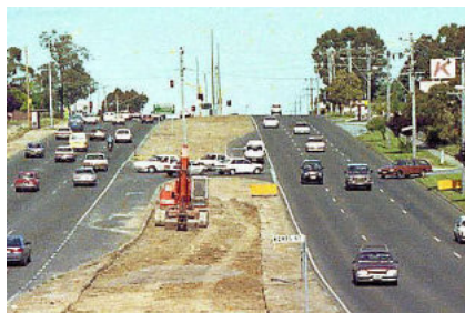
ABOVE: Burwood Highway looking east to Blackburn Road during earthworks (16 November 1992).
