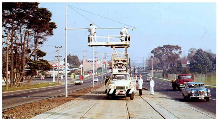
RIGHT: Installing trolley wire to booms adjacent to Burwood Primary School and PLC (June 1978).
