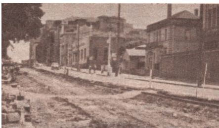
1963 reconstruction of the northern side of Victoria Parade, between Brunswick Street and Smith Street. Part of the cable tram lines can be seen at the edge of the work. From the February 1963 issue of Royalauto , in the collection of the Melbourne Tram Museum.
