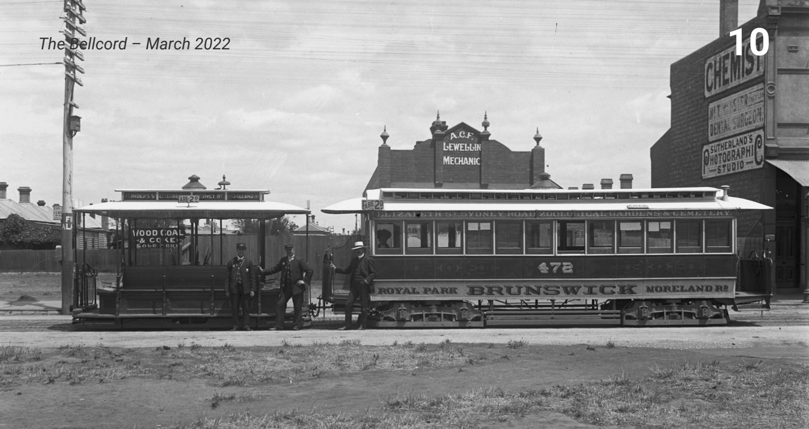
MTOC cable tram, Sydney Road, Brunswick, c1910. Photograph by C.A. Ratten, in the collection of the Melbourne Tram Museum.
