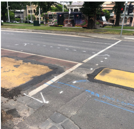
Markings denote the site of the cable tram pit in Victoria Parade, 9 January 2022. Photograph by Warren Doubleday.
