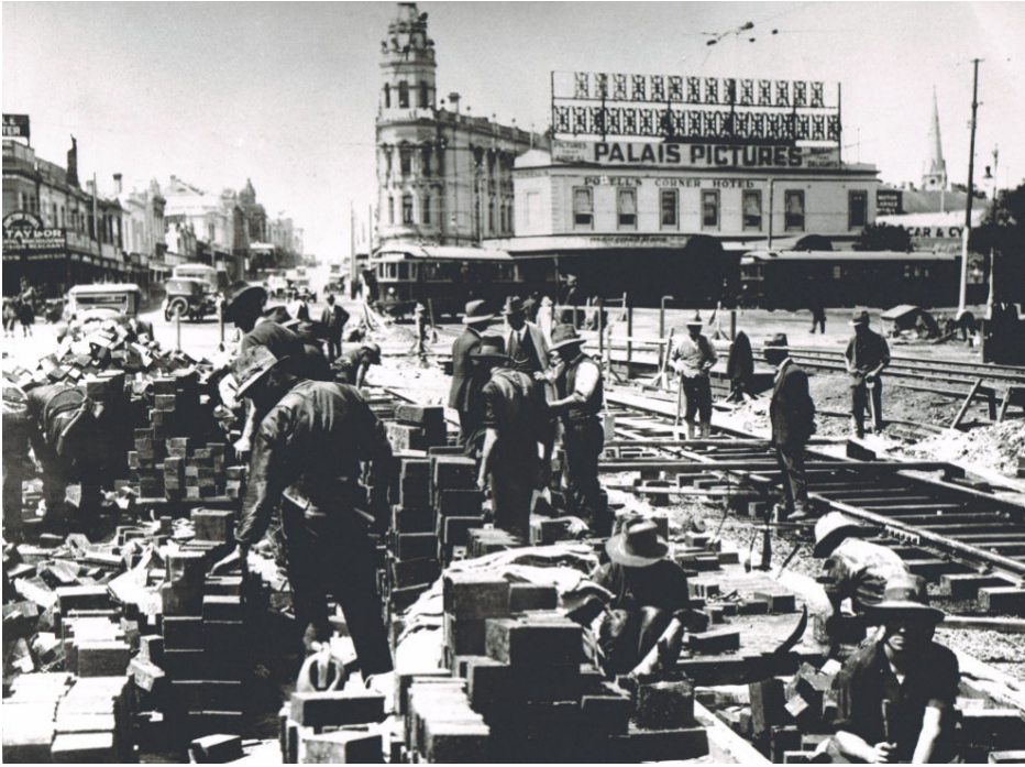
Woodblocks in the foreground during the reconstruction of St Kilda Junction in the 1920s as part of the conversion from cable to electric trams. Photograph from the collection of the Melbourne Tram Museum.
