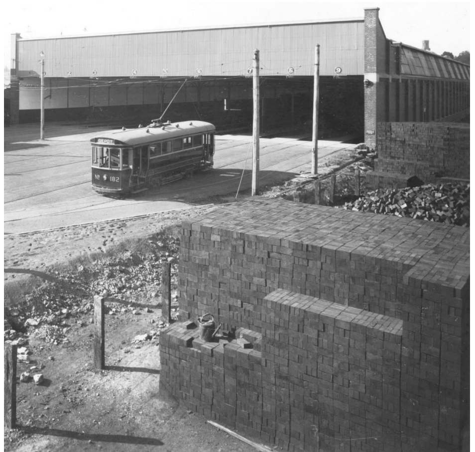
This photo dates from the early days of the Hanna Street Depot – late 1925 or early 1926. Cable tramways were being converted to electric tramways – including in Swanston Street and St Kilda Road. The piles of woodblocks are truly awesome! Photograph from the Ray Pearson collection, Melbourne Tram Museum.
