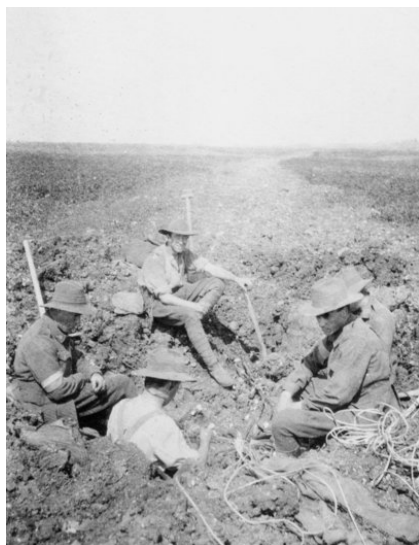
Members of the Second Divisional Signals Company east of Amiens, France, 1918, where they are repairing a broken or faulty telephone cable. The shallow trench they have dug gives little protection from enemy fire. Image courtesy of the Australian War Memorial.
