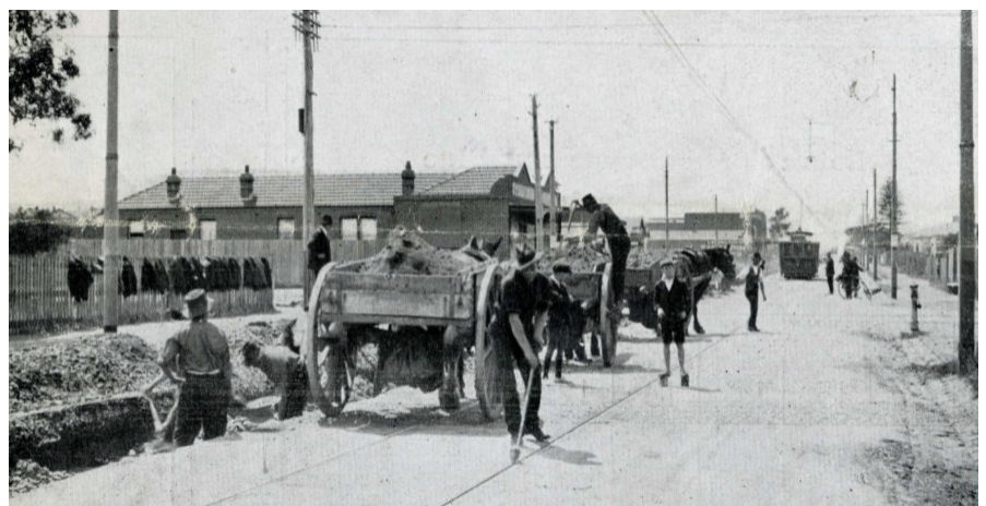
Duplication of the tram track at the corner of Glen Huntly and Bamba Roads, February 1923. The tram in the background is an early PMTT California combination car. Photograph from a real estate poster targeting tramway employees, from the collection of Len Millar.
